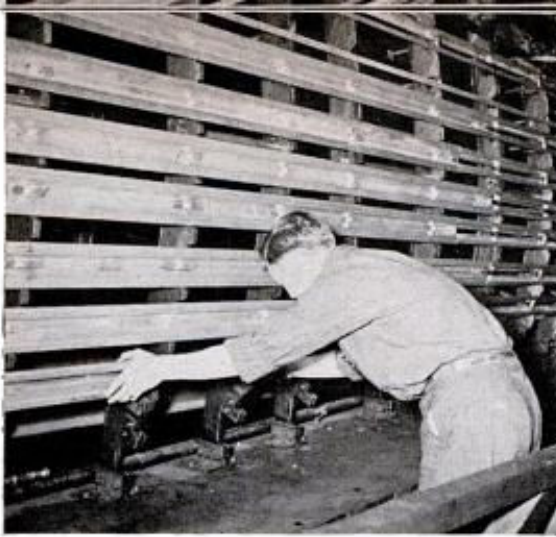
11 In another fixture, stringers are put in position for attaching to the wing skin. The stringers have been assembled so that they are lighter toward wing end (right)
