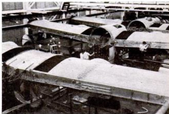
26 Now the Liberator really starts to take form. At the first mating station, bulkheads, longeron bomb racks, and side panels are installed. At the second, the nose is attached to the center wing. The stream flows on
